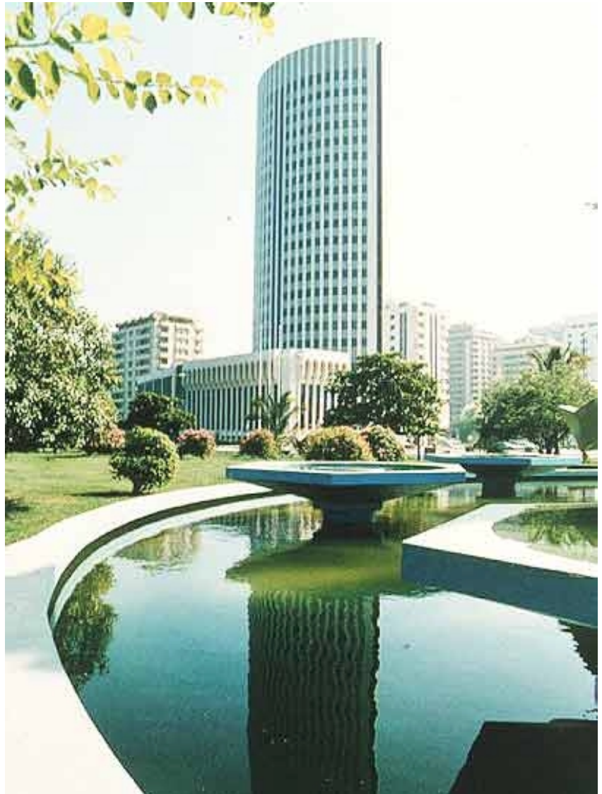
Construction of 22-storey elliptical tower on 4-storey podium.
